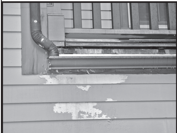
Above: 4. Synthetic siding showing some evidence of water infiltration.
