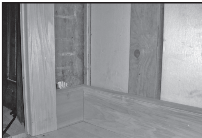
Rigid insulation cut to fit can be used where reversibility is a consideration Photo courtesy of the author.
