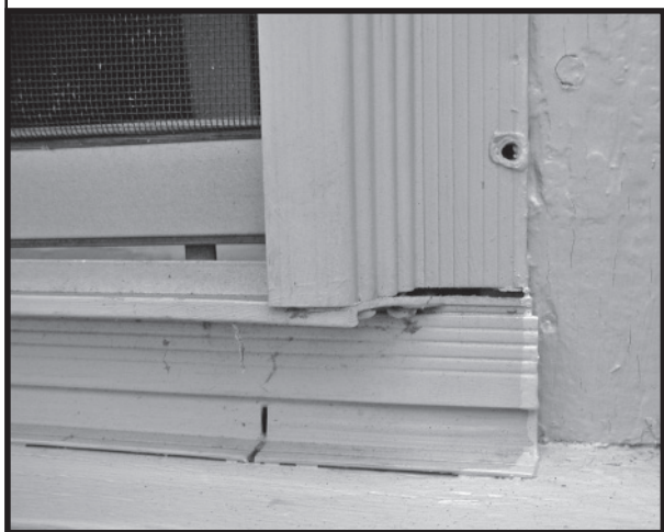
An ineffective storm window installation, allowing excessive air to move through the joints Photo courtesy of the author.
