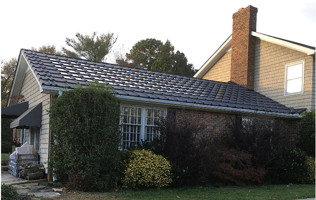
A DeSol Power Tiles installation.
