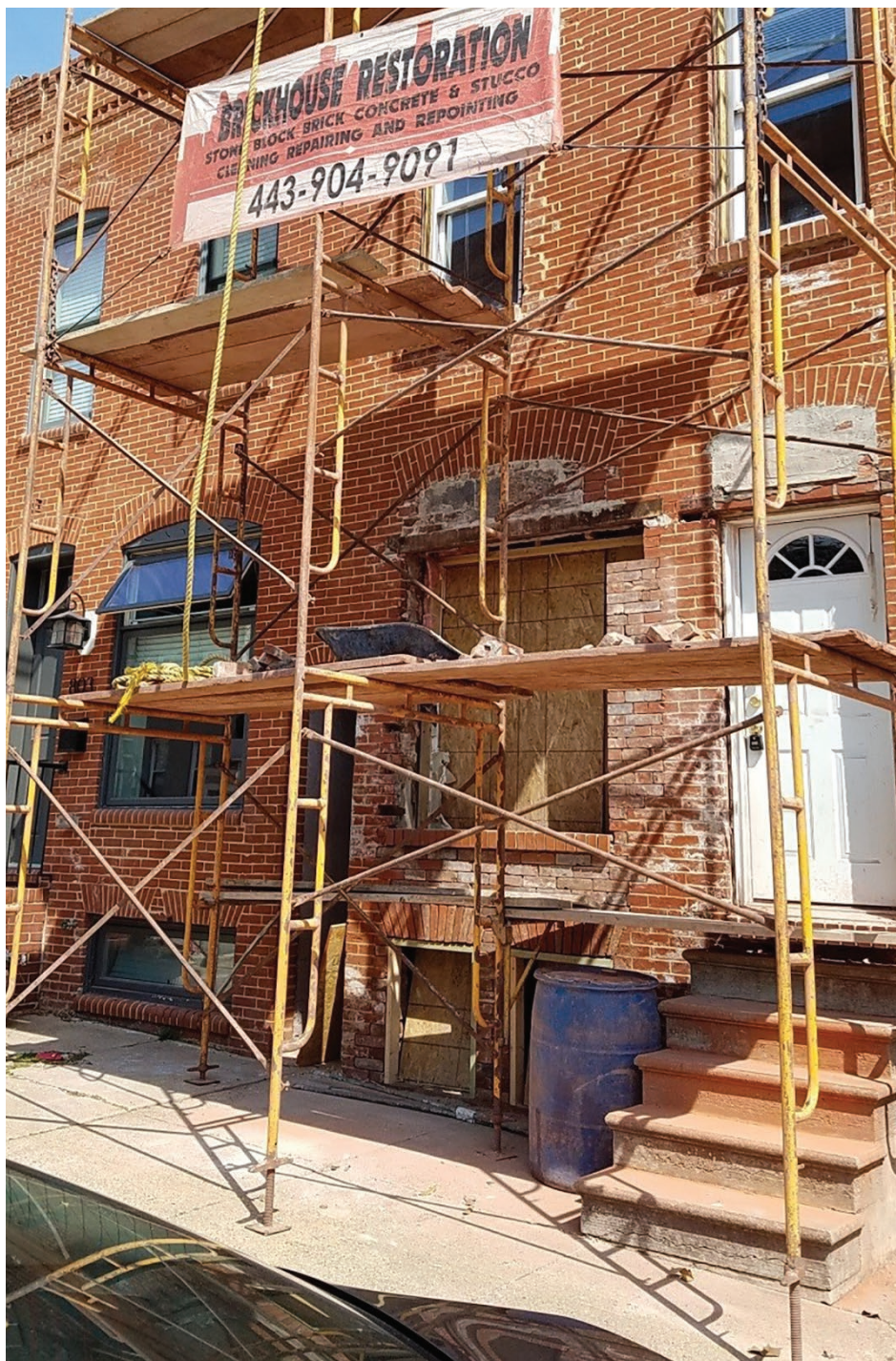
Example of Formstone removal and the restoration of the original brick surface at 805 S. Milton Avenue.
