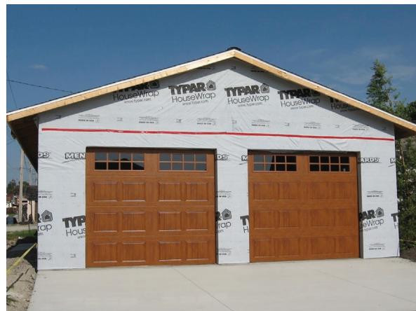
Example of appropriate overhead track metal doors on this new garage.
