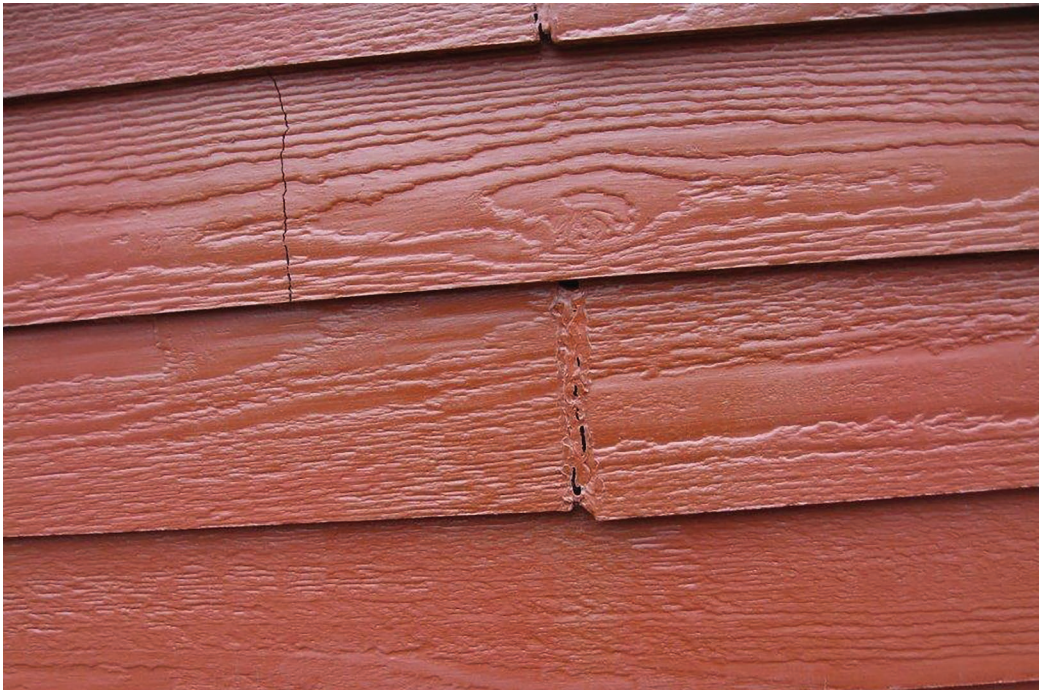
Fiber cement siding (one common trade name is HardiePlank) showing a false wood grain.
