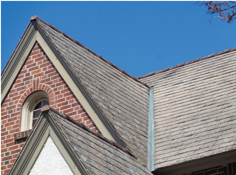
Numerous roof ridges with asbestos ridge tiles.
