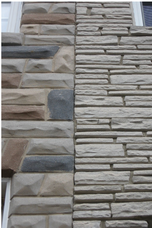
Formstone came in a variety of textures and colors as seen in these houses in Little Italy.
