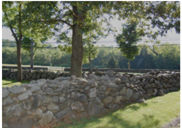
An example of a traditional dry-laid fieldstone wall, and a rehabilitated wall in the background-all using local stone.
