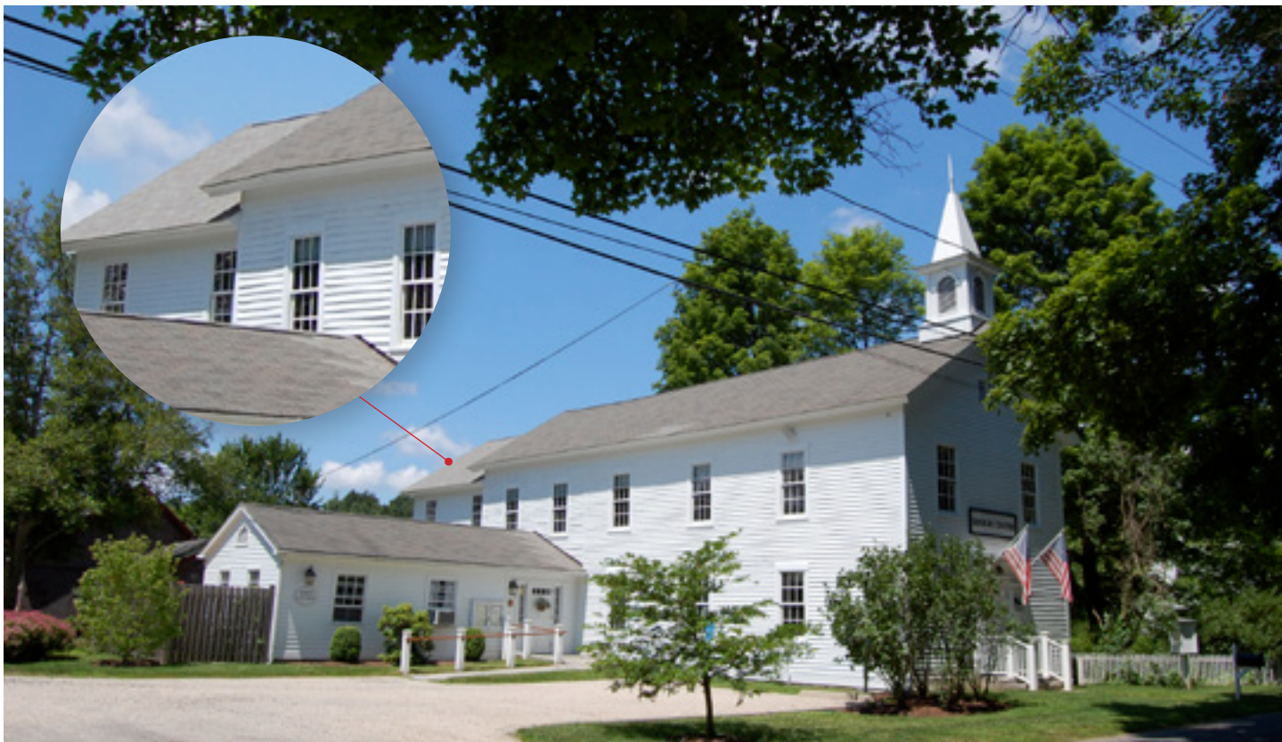
The new addition to the Old Town Hall, now the Senior Center (west, rear) is differentiated from the historic building by a setback in the roof and plane of the building.
